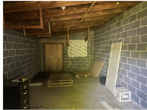
Interior of building before work began
